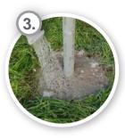
For larger foundations such as street furniture, swings, clotheslines, etc., the size of the hole should be approximately 30 cm on each side and 40 cm deep. Apply the product in two successive layers of 20 cm fresh on fresh.
